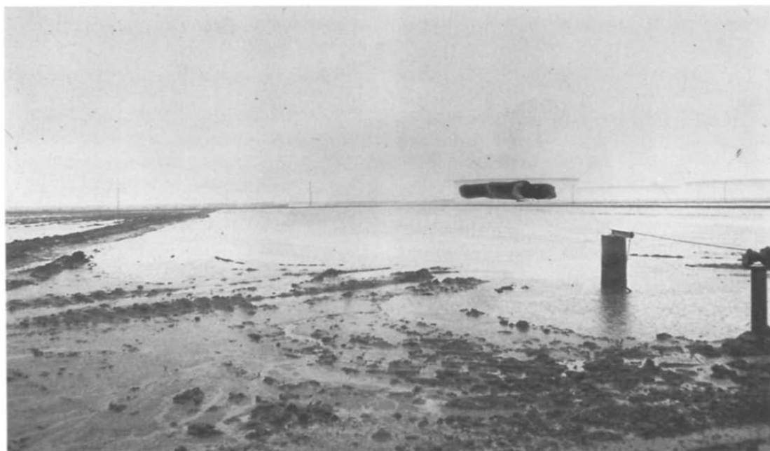
Fig. 3. Oily residue prior to filtration.
